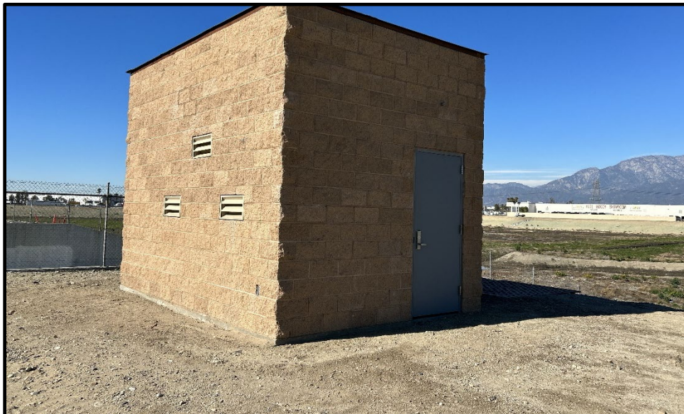
Wineville Basin – Rubber Dam Building (Completed Building Structure)
